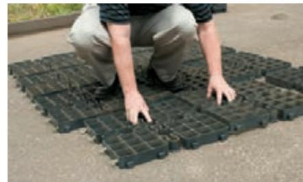
**How to expand the Core Buster Drag Mat****To add an additional vertical row:**
